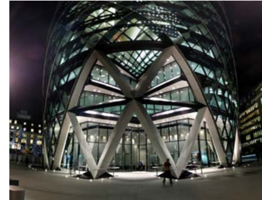
Above: Gherkin Tower, London The tower base has no area for commercial activity.
