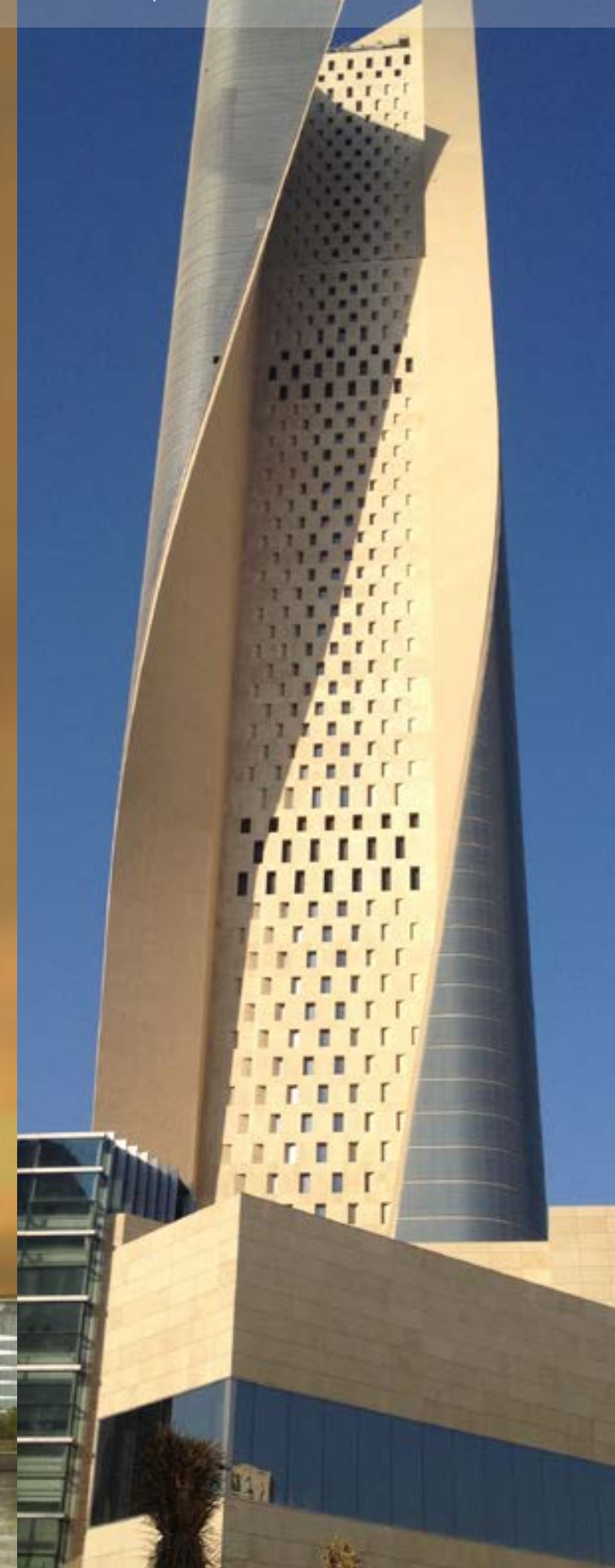
Al Hamra Tower Kuwait City
