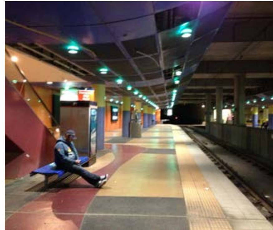
Existing Light Rail Station
